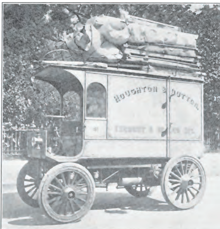
The Horseless Age , October 29, 1902, included a picture of the large, 1-½ ton capacity commercial delivery wagon Upton had built for a Boston department store. It had an opposed two-cylinder, twenty horsepower engine coupled to a larger planetary transmission with a chain drive to the rear end. The Upton Machine Company manufactured the frame, engine, transmission, and rear end in their facility. It is unknown if the body was built in-house or by a local shop.
